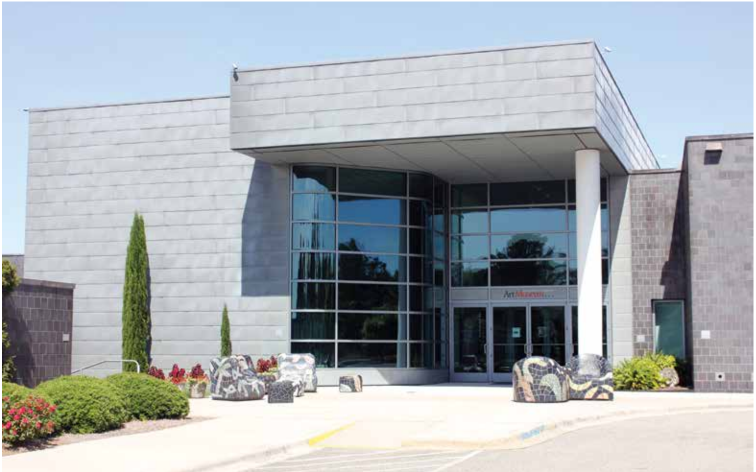
Completed in 2002, the Cameron Art Museum was designed by architect Charles Gwathmey with a ventilation system inside the masonry that allows the building to “breathe” during hurricanes, which are a feature of life in Wilmington, North Carolina.
