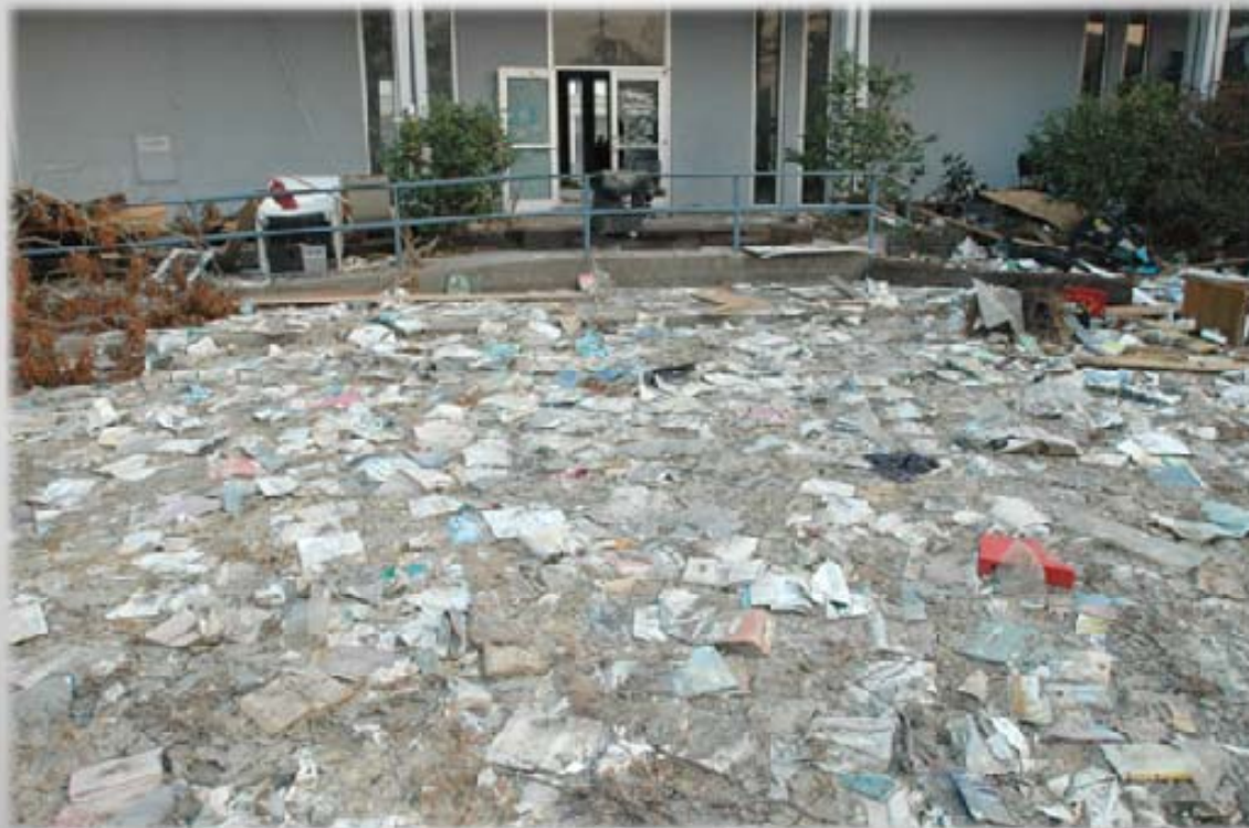
Hurricane Katrina damage Pass Christian Public Library, Mississippi FEMA/Mark Wolfe
