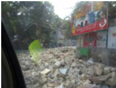
In some area, building debris narrows the street
