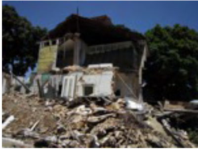
Damaged Center D'Art building
