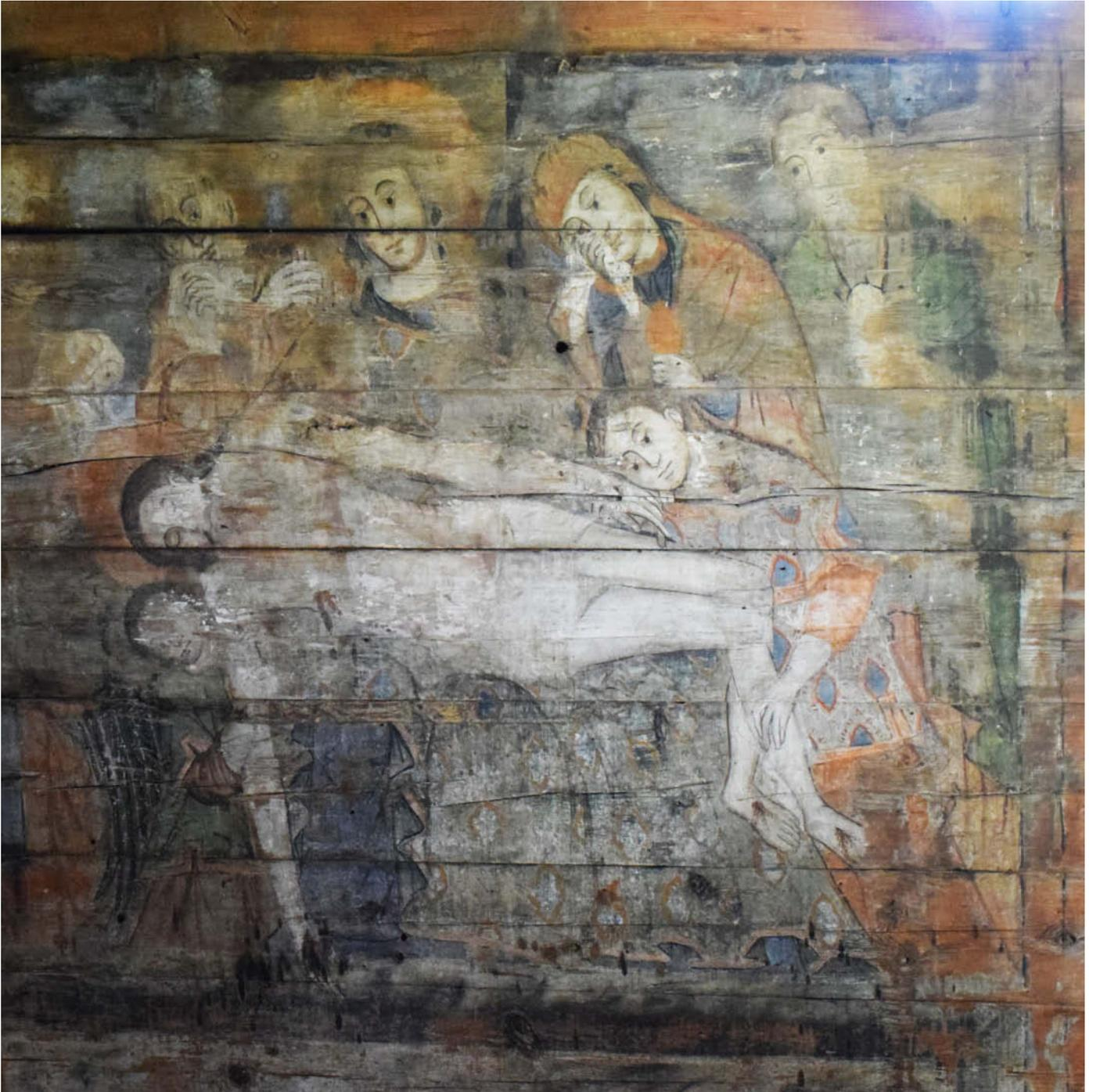
Fig. 2. Paint losses, interior timber walls, Tserkva of the Descent of the Holy Spirit, Potelych, Ukraine, ca. 1502.
