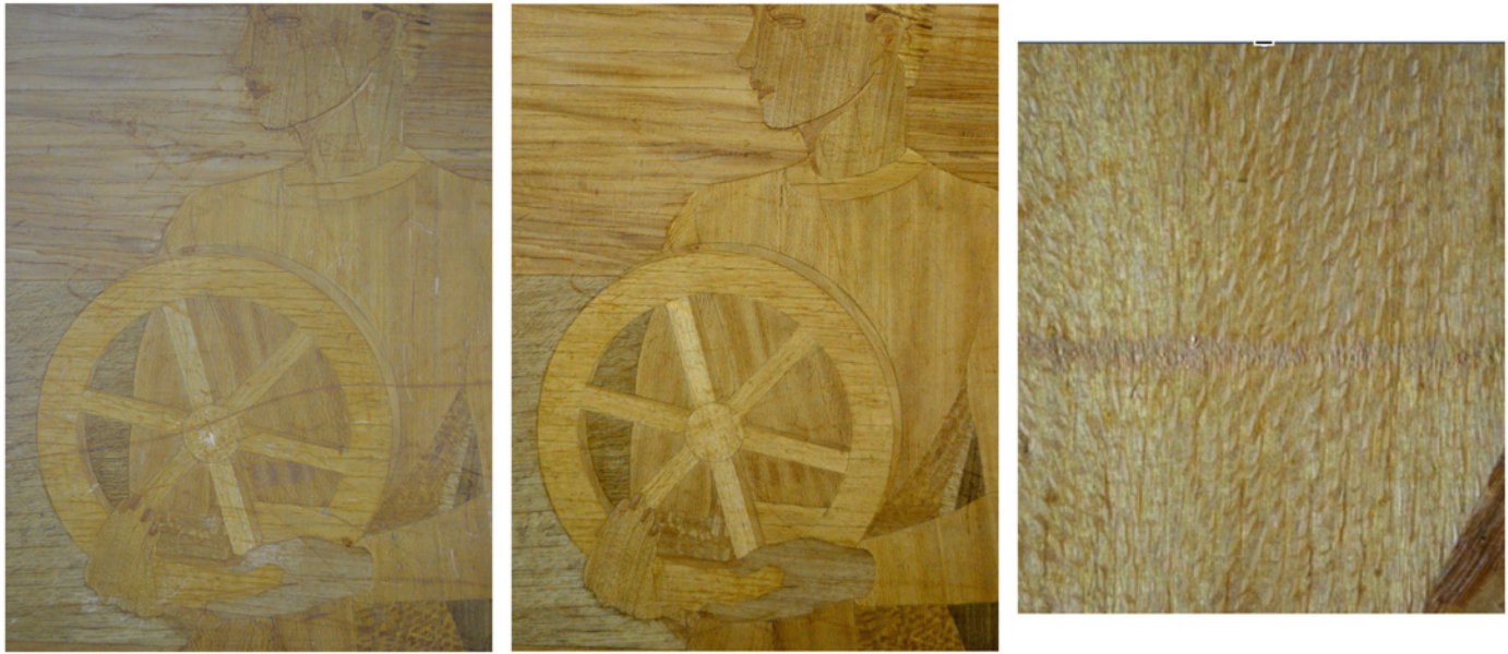
Fig. 18. Left: Detail before and after images of the lower right panel with mitigation of darkened scratches. Right: Detail of use of mica powders to retouch darkened scratch.
