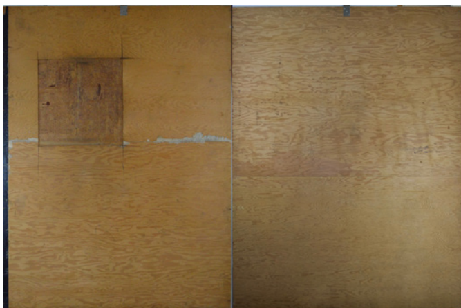
Fig. 8. Backsides of two side marquetry panels showing Douglas fir plywood.
