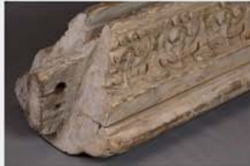
Fig. 2 Whitish haze on exposed and unexposed surfaces on a section of a pine handrail
