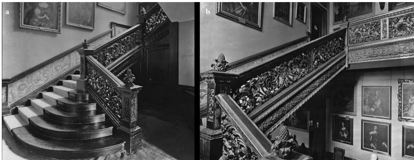
Fig. 2. Staircase after it was reinstalled at Cassiobury House at the beginning of the 19th century. a. Lower long flight with the bottommost five steps opened up to provide a grander entrance; b. Balustrades of the short flight, the upper long flight, and the upper floor (©Victoria and Albert Museum, London. 'Cassiobury Park file, Furniture, Textiles and Fashion Department, V&A'. Unidentified print)
