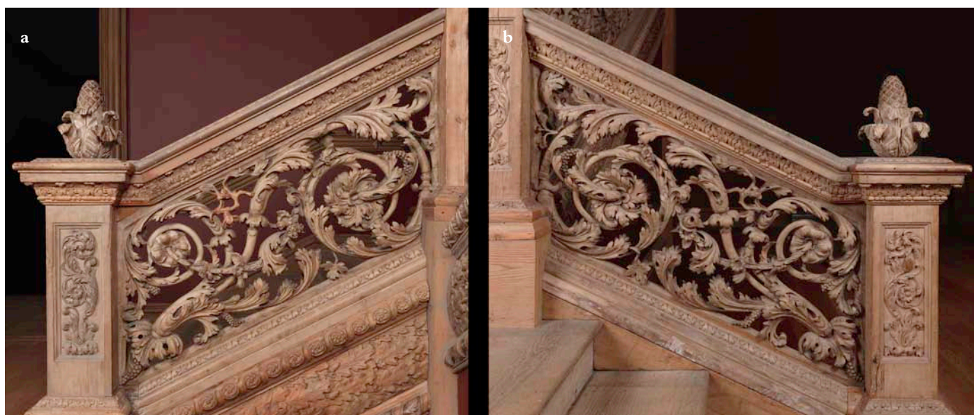
Fig. 3. Balustrade of bottom short flight (BT). Three different types of wood were used for the creation of the staircase: elm for the pierced and double-sided carved baluster friezes, finials, and pendants; oak for the steps and landings; and pine for everything else. a. Exterior side; b. Interior side. (© The Metropolitan Museum of Art)
